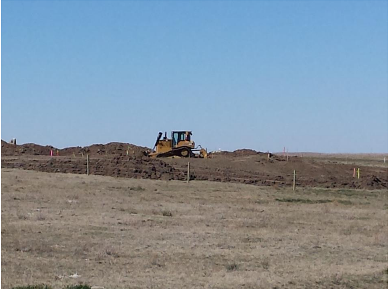
Figure 4. Reclamation activities on an abandoned lease. Photo Shannon Burnard.
